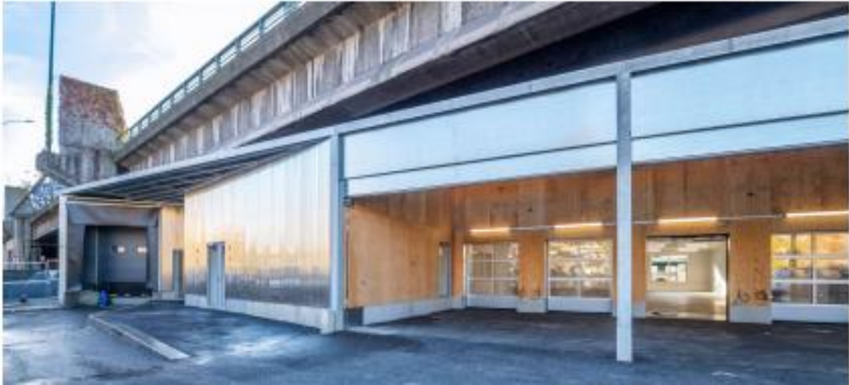
Figure 1: P4 site - 19th arrondissement of Paris. Winner of the MIPIM 2021 award. Source: Sogaris
