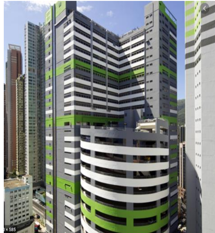
Goodman building in Hong Kong (24 levels)
